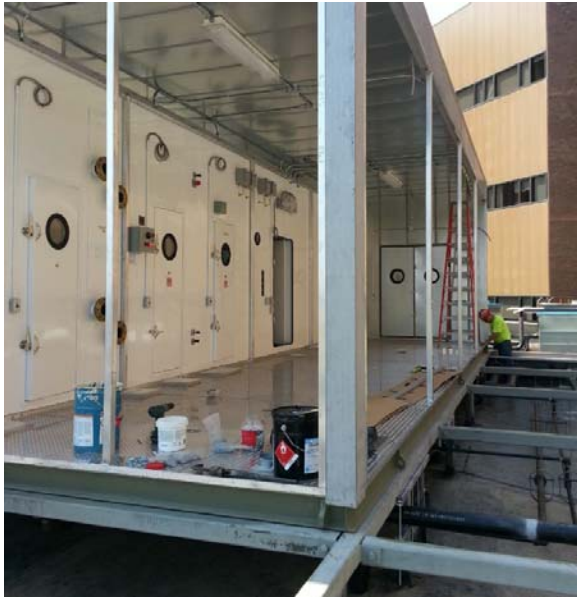
(Above) The first two sections of AHU-37A are shown on its base. Section One contains the heating and cooling modules, followed by a humidifier, silencer, fans and final filters. Section Two is the service vestibule.
