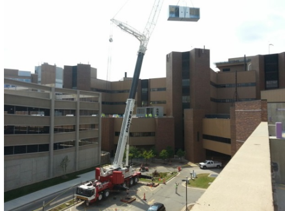
(Above) The final section of AHU-37A, shown as it was lifted into place.
