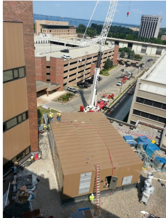
(Above) The four sections of the unit are shown fully assembled and awaiting louvers.
